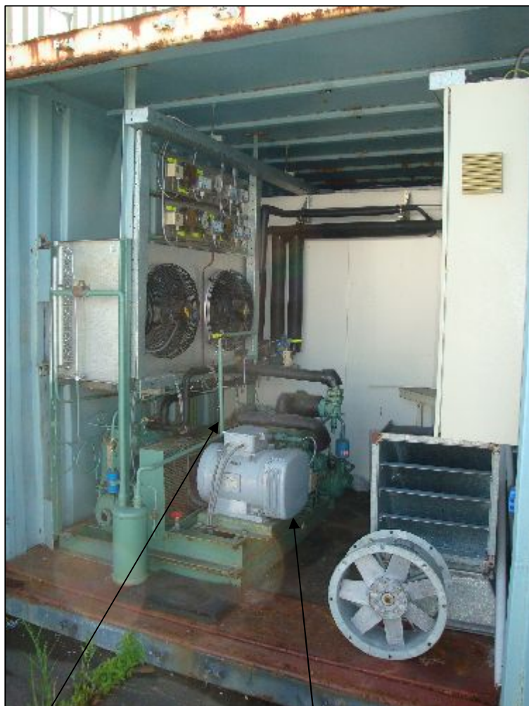
Bitzer compressors Leroy Summer E Motor 18.5 kw
